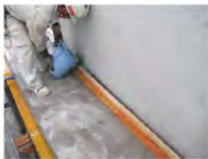
(h) Fiber mortar for wall bed
