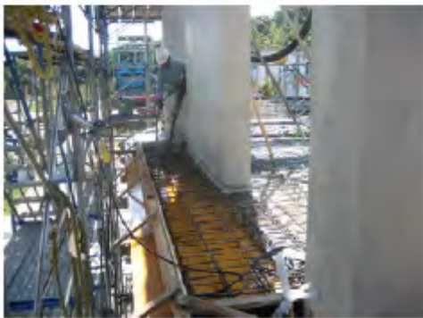
(c) Concrete cast around wall
