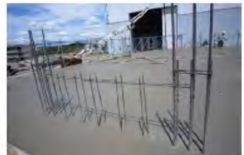
(g) Concrete cast
