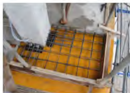
(h) Steel arrangement for corner slab
