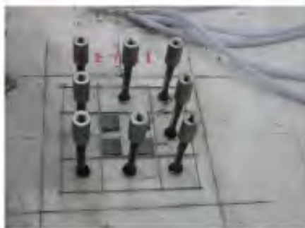
(c) Threaded couplers above foundation
