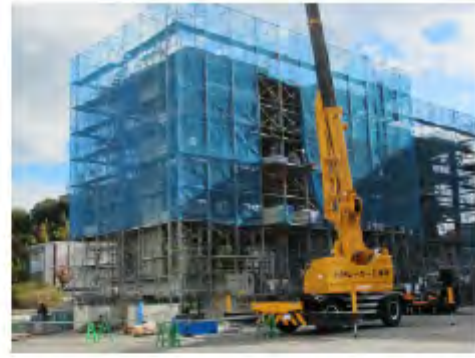
(e) Preparation for prestressing the multi-story wall
