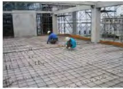
(e) Steel arrangement for top slab
