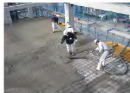
(f) Cast of top concrete
