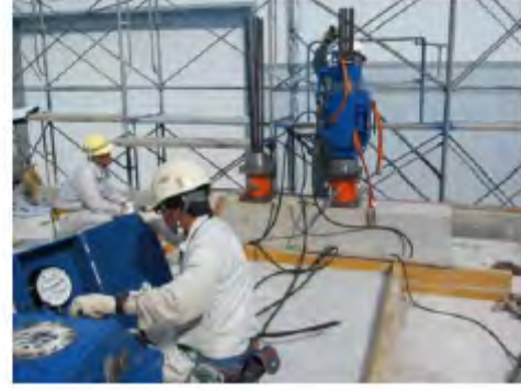
(g) Pump and jack prestressing PT wire
