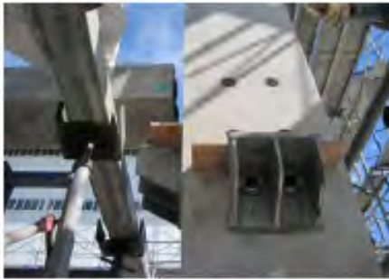
(b) Bracket supporting beam end
