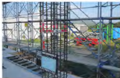
(c) Steel arrangement of column
