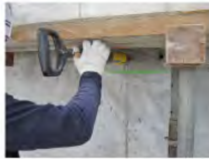
(e) Grouted coupler (injection of mortar)
