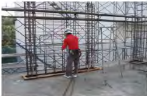
(b) Steel arrangement of wall
