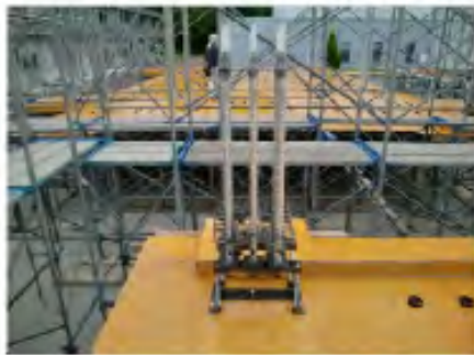
(a) Anchorage of PT bars in foundation
