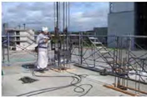
(a) Gas pressure welding
