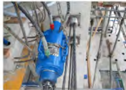
(g) Beam prestressed after concrete cast
