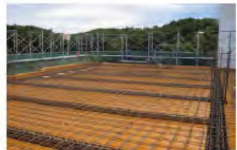
(f) Floor placing steel bars
