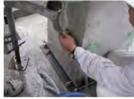
(g) Grouted column bed (mortar)
