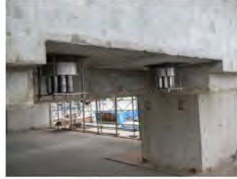
(f) Anchorage of PT wires beneath foundation
