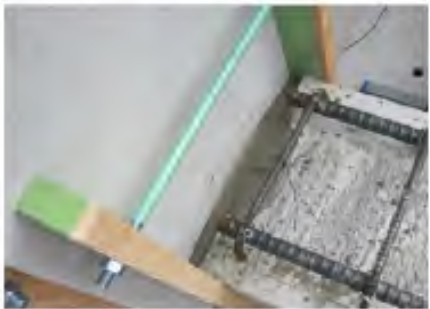
(c) Grouted beam end (mortar)
