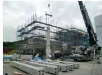
(e) Lift-up of the precast concrete column
