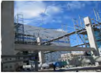
(a) Placing half precast concrete beam
