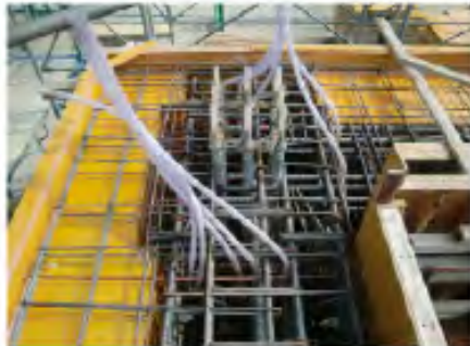
(b) Steel arrangement of foundation
