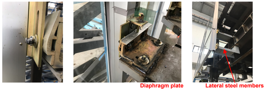
Figure 4. Photos of fasteners fixed at the diaphragm plate or lateral steel member
