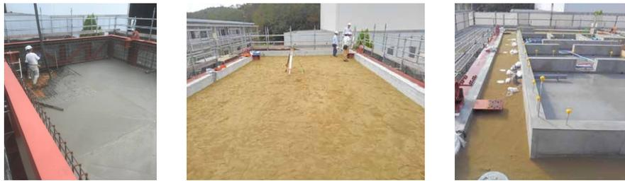
(1) Reinforced concrete soil box (2) Compacted soil (3) Foundation constructed on the soil
