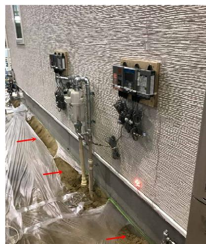
(2) Bent polyethylene gas pipes
