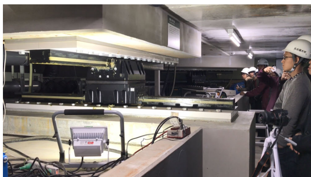
FIGURE 5. Observation of the base-isolated layer of the seismic building.
